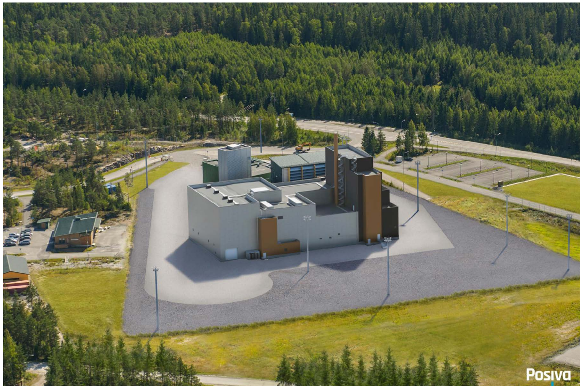
FIGURE 21. The encapsulation facility of Posiva (Posiva Oy).
